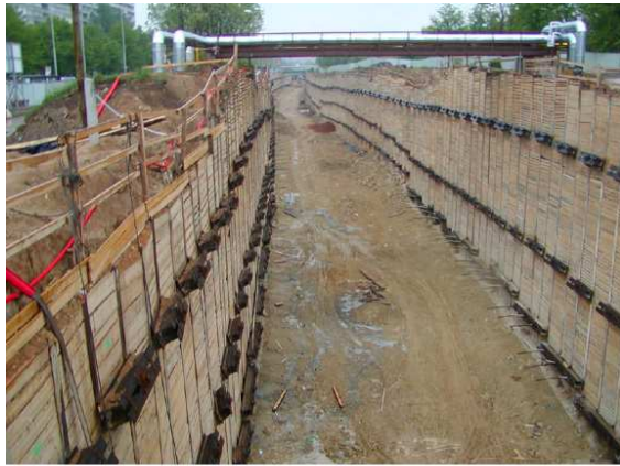
Fig. 1 Open pit for the cut-and-cover tunnels between the Střížkov and Prosek stations
