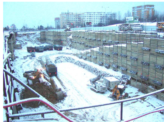
Fig. 5 Temporary ramp
