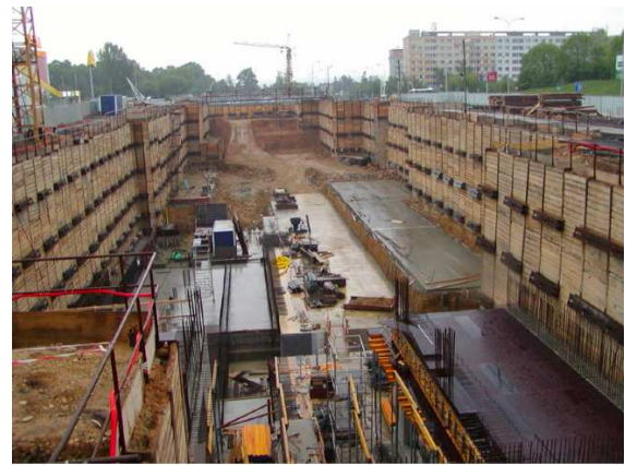
Fig. 3 Prosek station - open pit
