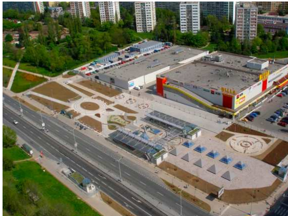
Fig. 2 Aerial view of the finished Prosek station
