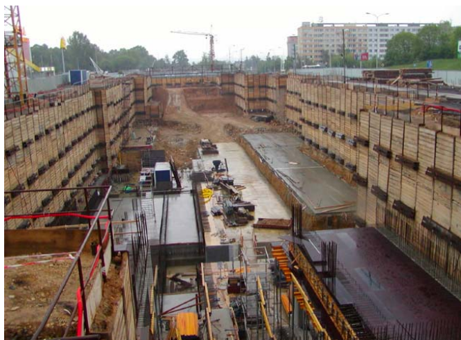
Figure 6 Prosek station – irregularly-shaped open pit
