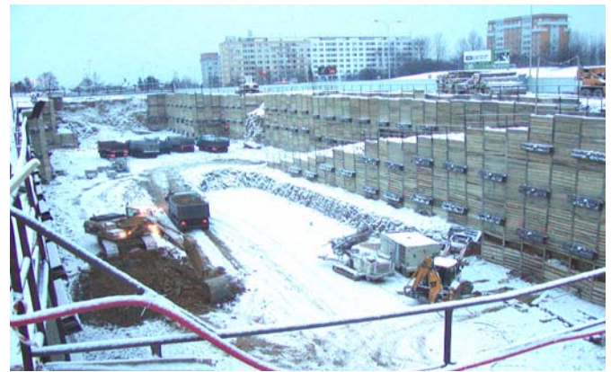
Figure 7 Temporary ramp in the open pit Prosek
