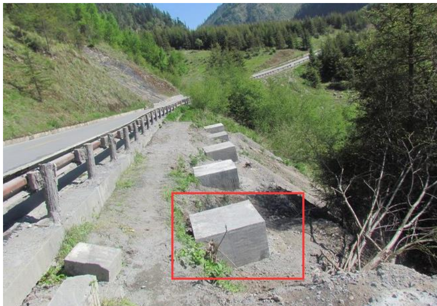
Anti-slide piles (all below the terrain)
